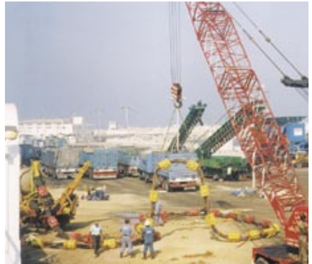
Bending control on umbilical bundle.
